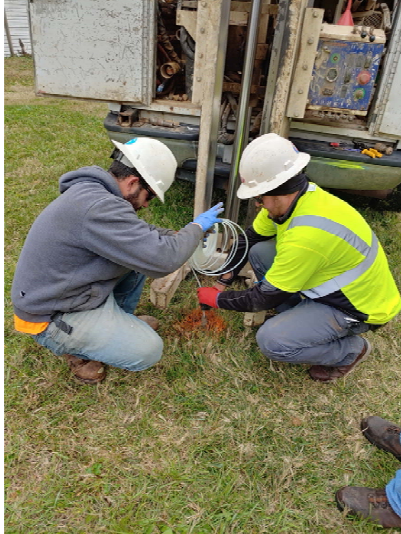
Soil vapor probes installation. Vapor inlet screen installed 15 feet below the surface. Flexible tubing attached to probe and extends to surface. Steel box and concrete pad constructed to protect tubing.
