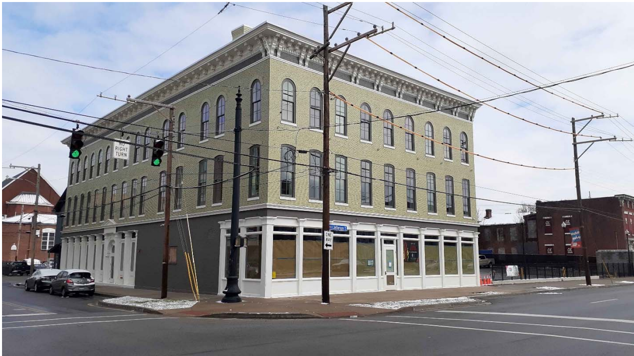
Hancock House (formerly Louisville Chemical Company) after renovation.
