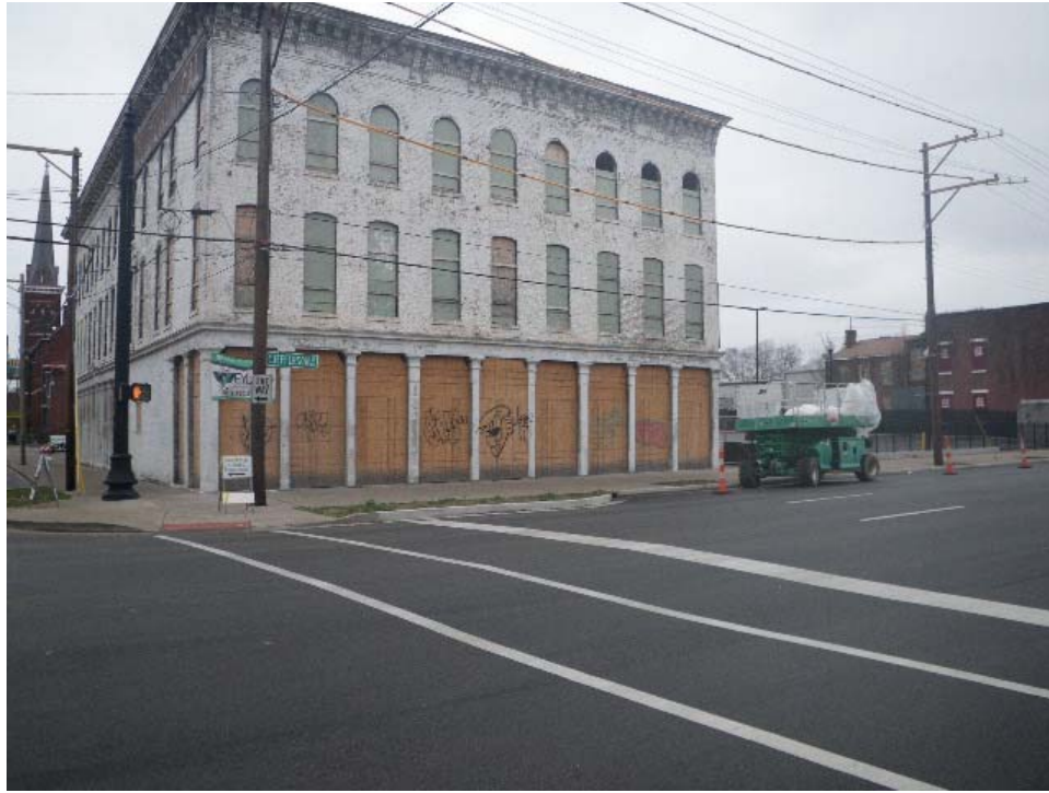
Former Louisville Chemical Company Building prior to renovation.
