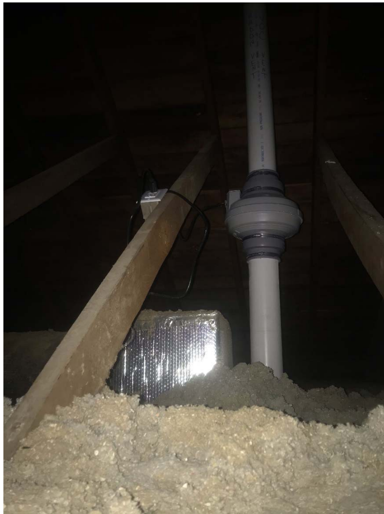
Leitchfield Cleaners -Vent line and vacuum routing vapors through the attic.
