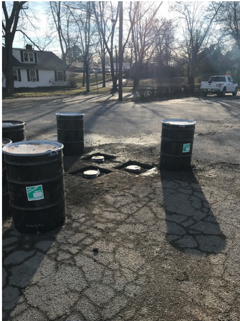
Nested Wells at Parrish Avenue to monitor three groundwater zones. Drums are cuttings to be disposed.
