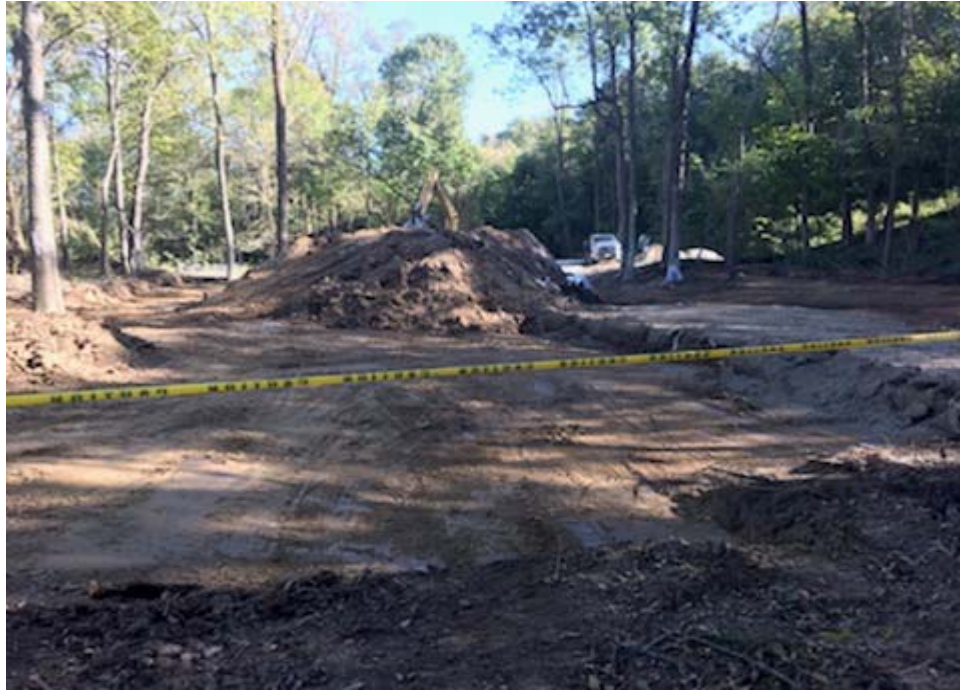
Stockpiling of soil in the pond area for soil amendment before removal.
